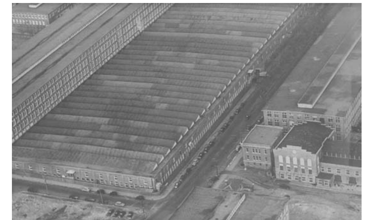
The building's unusual saw-toothed roof allowed more natural light to enter the manufacturing area.
